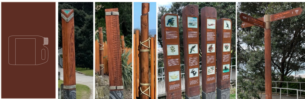
Figure 6: The Abodo Waterborne Protector Oil (Manuka) paint colour (suppliers sample on left) used on Mauao can vary considerably depending on the wood being used.
